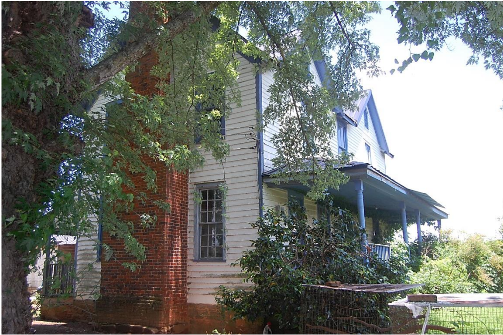
Jones-Waldrop House, Façade and Side (West) Elevation, Looking East.
