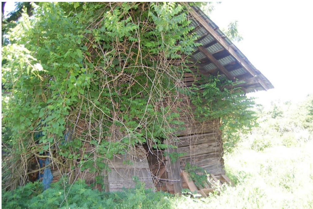
Jones-Waldrop House, Ruinous Log Smokehouse, Looking East.
