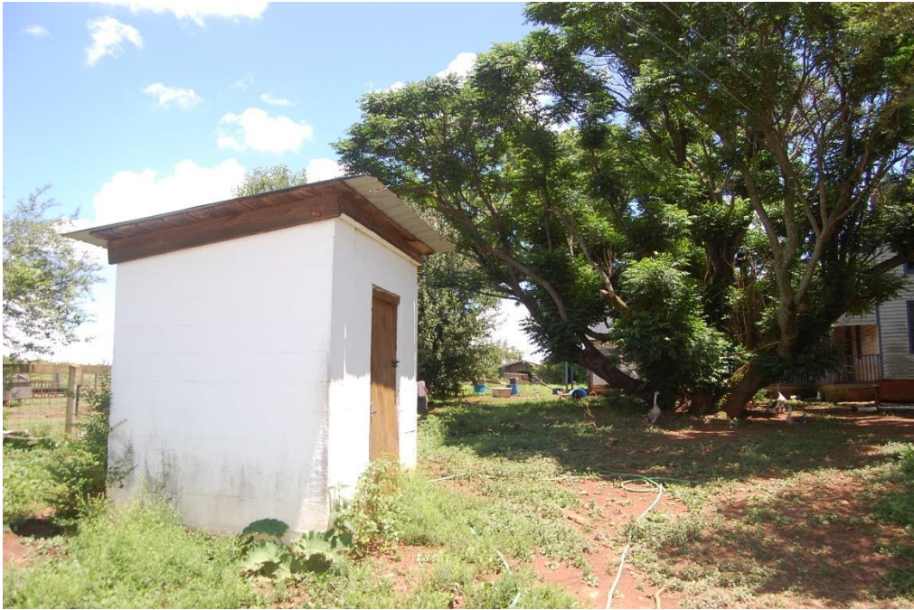
Jones-Waldrop House, Concrete-Block Pump House, Looking East.
