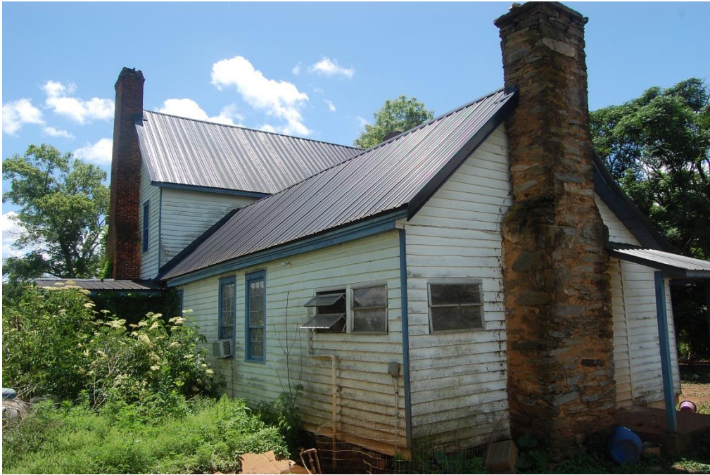
Jones-Waldrop House, Rear Kitchen Wing, Rear (North) and Side (East) Elevations, Looking South.
