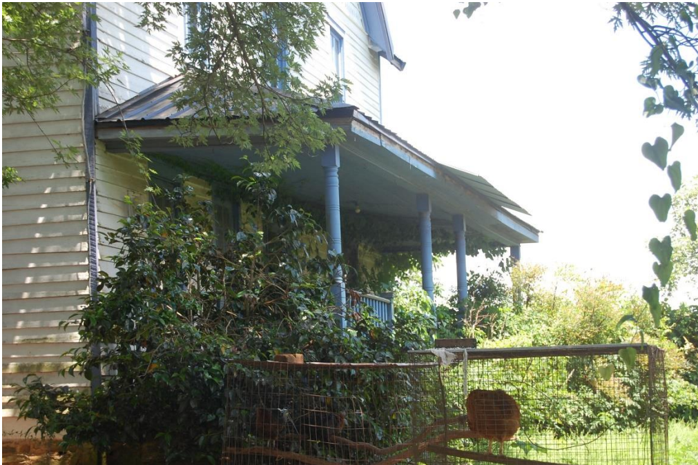
Jones-Waldrop House, Front Porch, Looking East.
