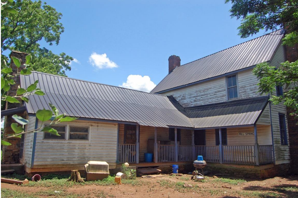
Jones-Waldrop House, Rear Kitchen Wing, Looking Southeast.
