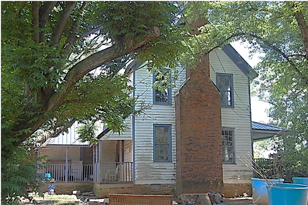
Jones-Waldrop House, Side (West) Elevation and Kitchen Wing, Looking East.
