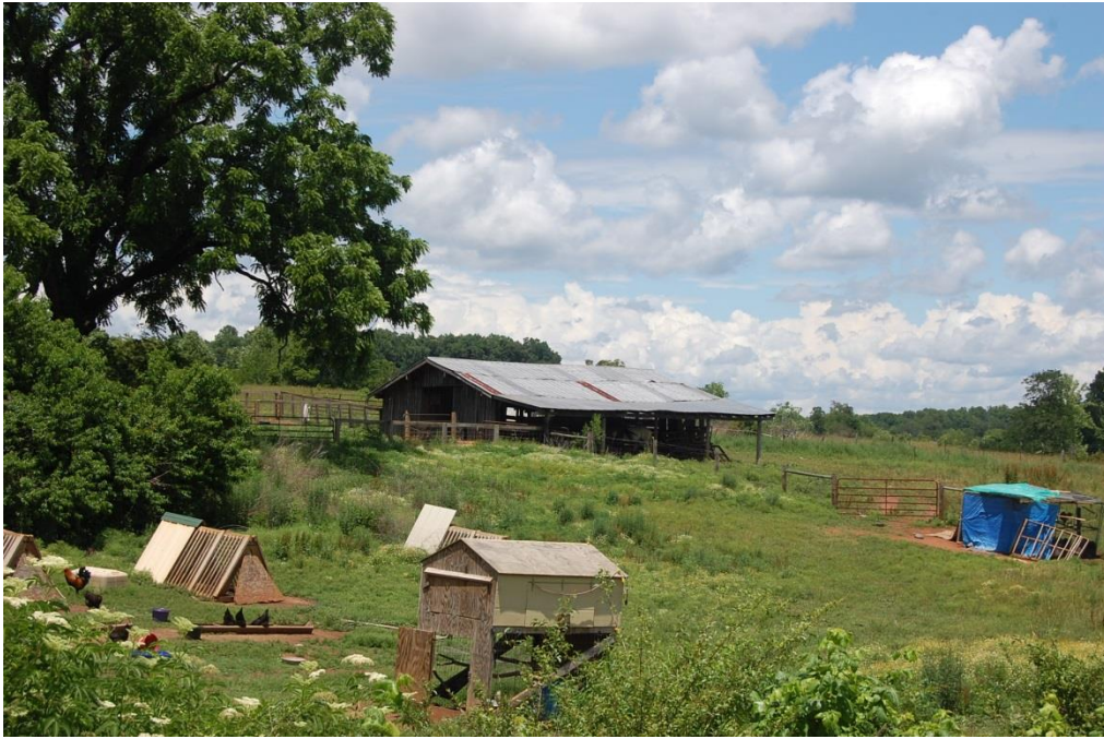
Jones-Waldrop House, Livestock Shelter (Poultry Pens in Front), Looking Northeast.
